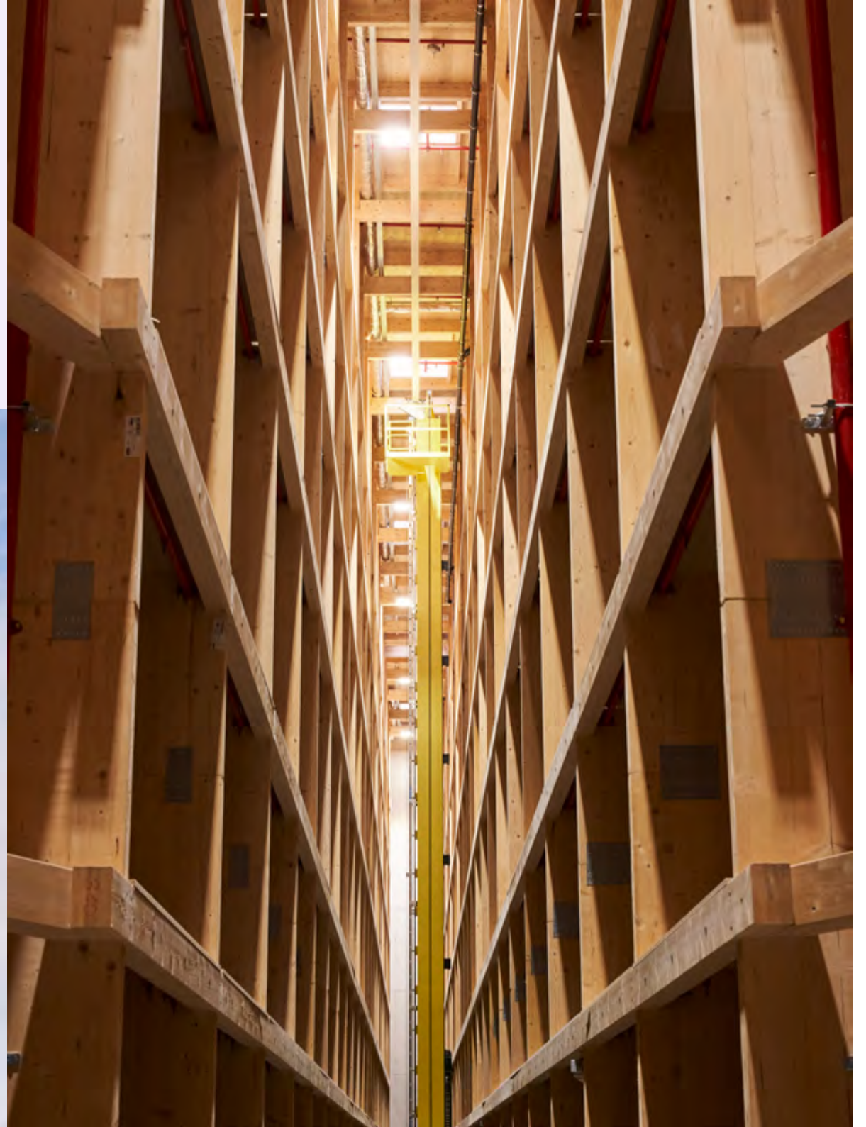
Wooden shelving with capacity for 17,000 pallets in the high-bay warehouse.
